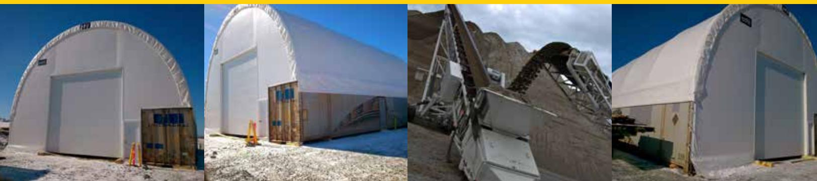
**“We chose the building from Britespan for its portability. The container foundation allows us to deconstruct and move the entire building to a new exploration site when we are finished.”**
