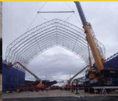
**The advantage of using the containers as a foundation for the structure was that the customer didn't have to purchase a wider building to achieve the height they required.**
