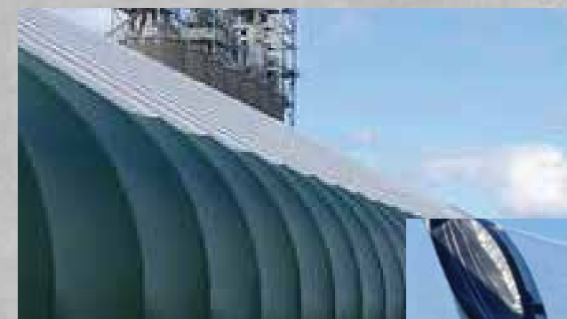
Round tube allows for proper tensioning without cover failure.
