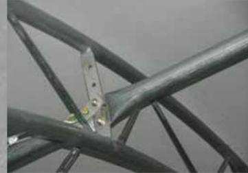
Britespan's standard double bolted solid purlin mount.
