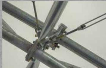
Britespan's standard solid bolted cable attachment.
