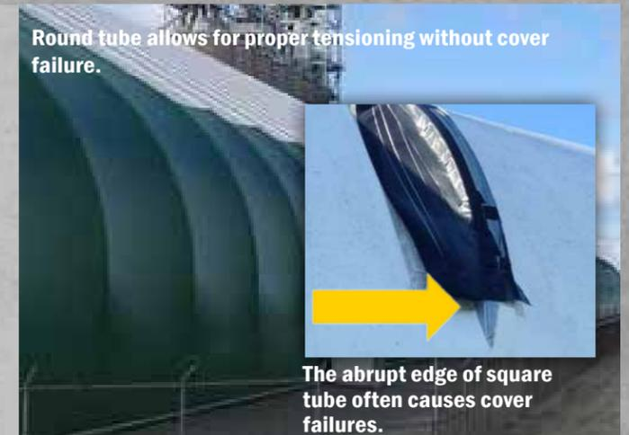
Round tube allows for proper tensioning without cover failure.
